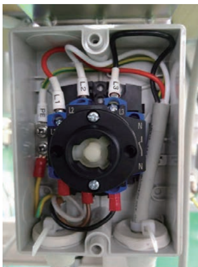
Power supply connection, 3-phase, 200-240 V
